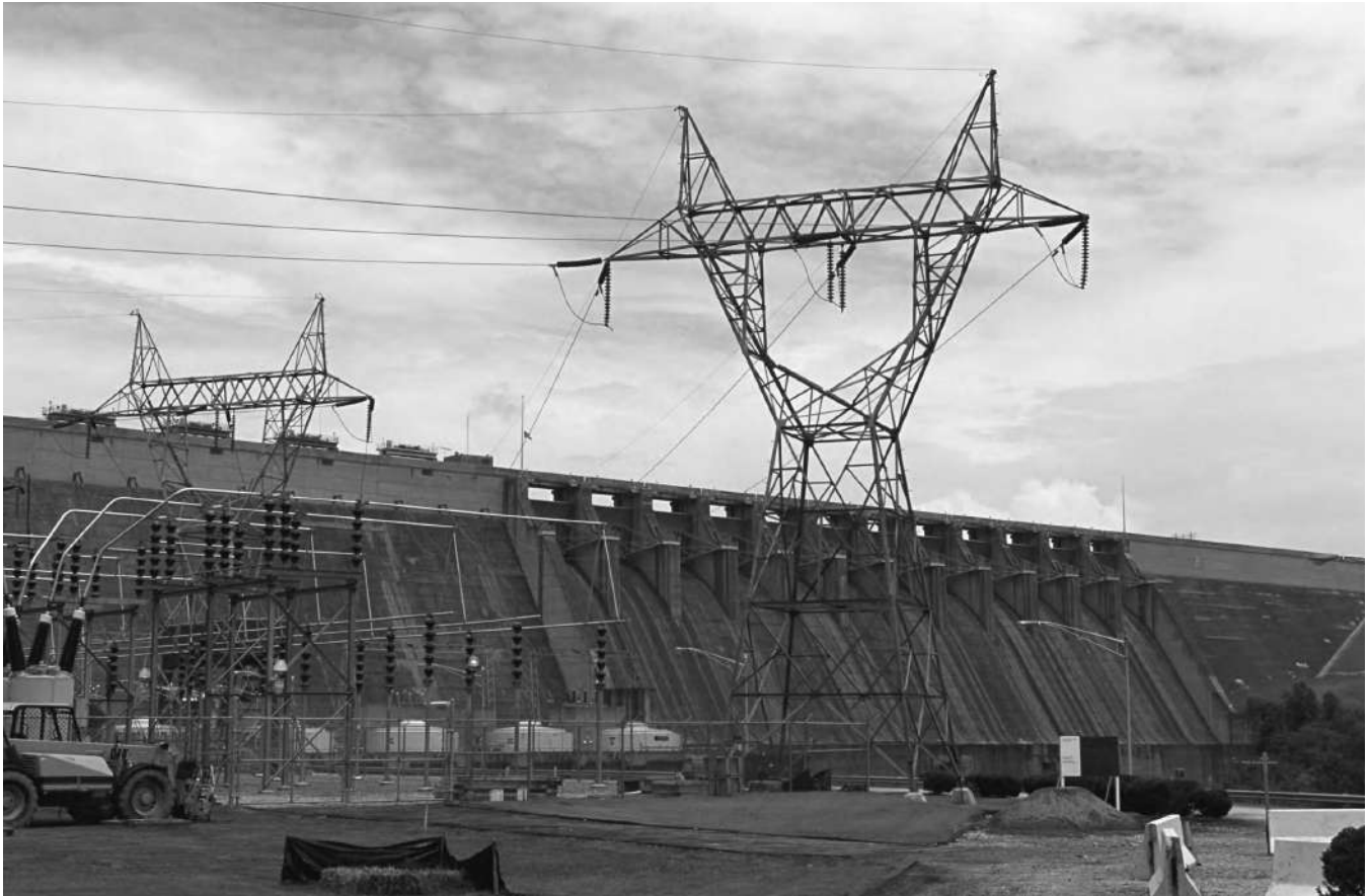
A hydroelectric plant in Tennessee. Once the water level reaches a high enough level, a gate is opened in the dam, allowing gravity to carry water down toward the generator. The force of the water falling spins the turbine and generator, creating electricity.
